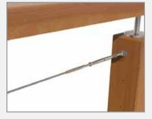
Lock the hex nuts against the body of the rigging screw to lock the system in place.
